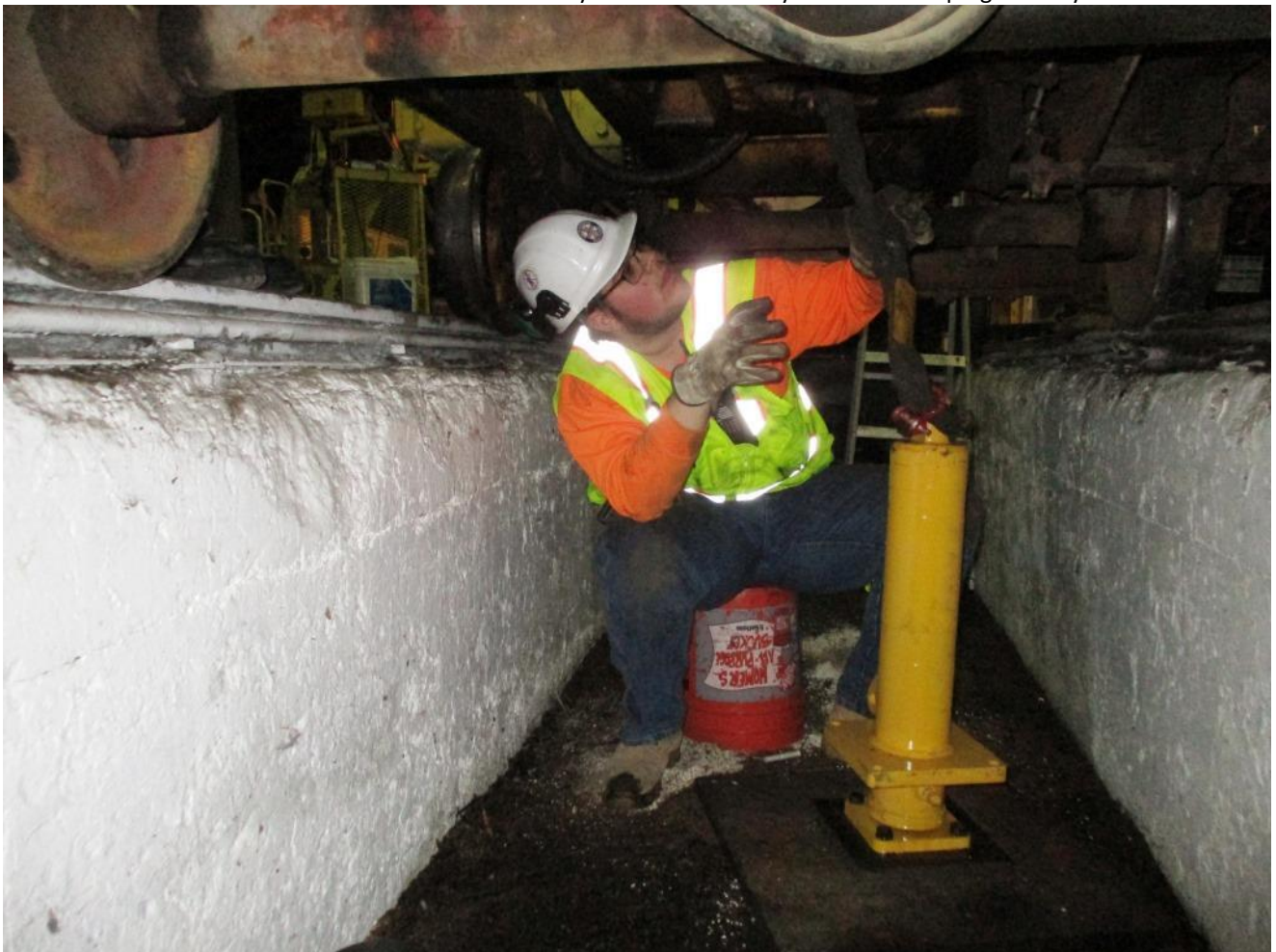
Chris H. in the pit under the 125 feeds the strap up through the engine compartment which will lift the cylinder into place
