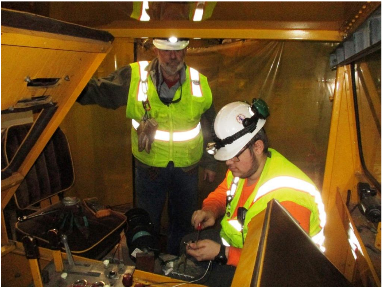
Art and Chris H. take care of the MT-14's electrical issues
